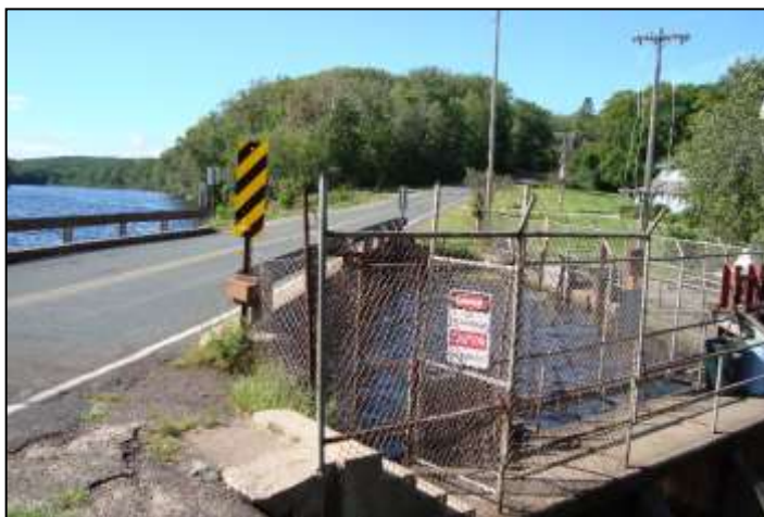
Clam Falls Dam and adjacent highway
