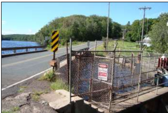
Clam Falls Dam and adjacent highway
